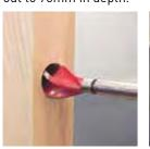
**Step two:** Using the same bit, drill the hole for the spindle.
